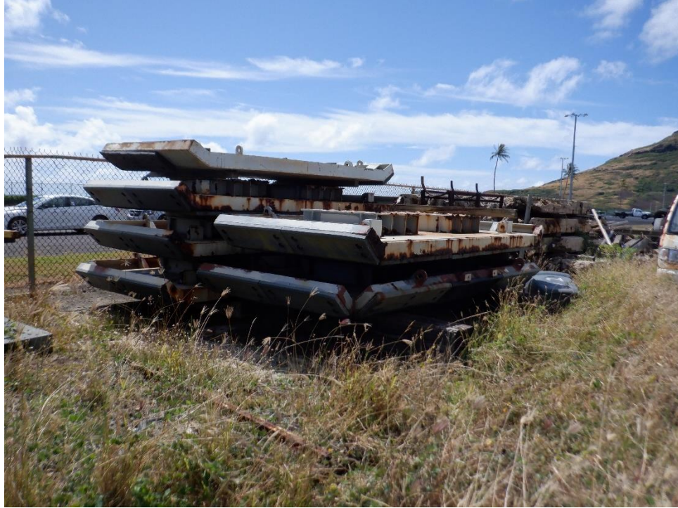
Photo 3: Fender Steel Frames for Removal and Disposal
