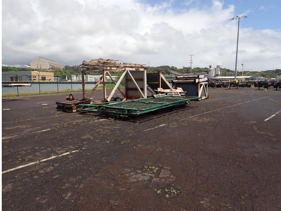
Photo 2: Additional Superferry Ramp and Chain Link Fence Components for Removal and Disposal
